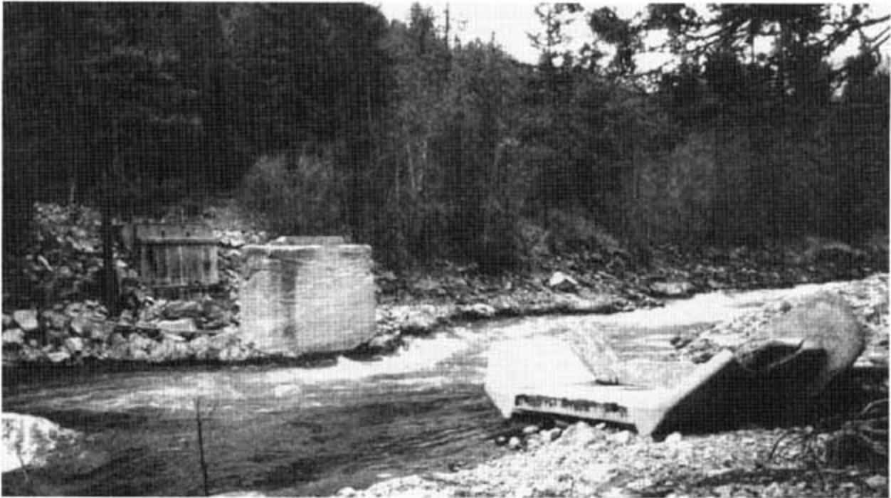
Figure 6. Eagle Creek Loop Road over Trinity River after flood of January 1, 1997. One pier wall is submerged. The standing pier and abutment walls are on bedrock.
