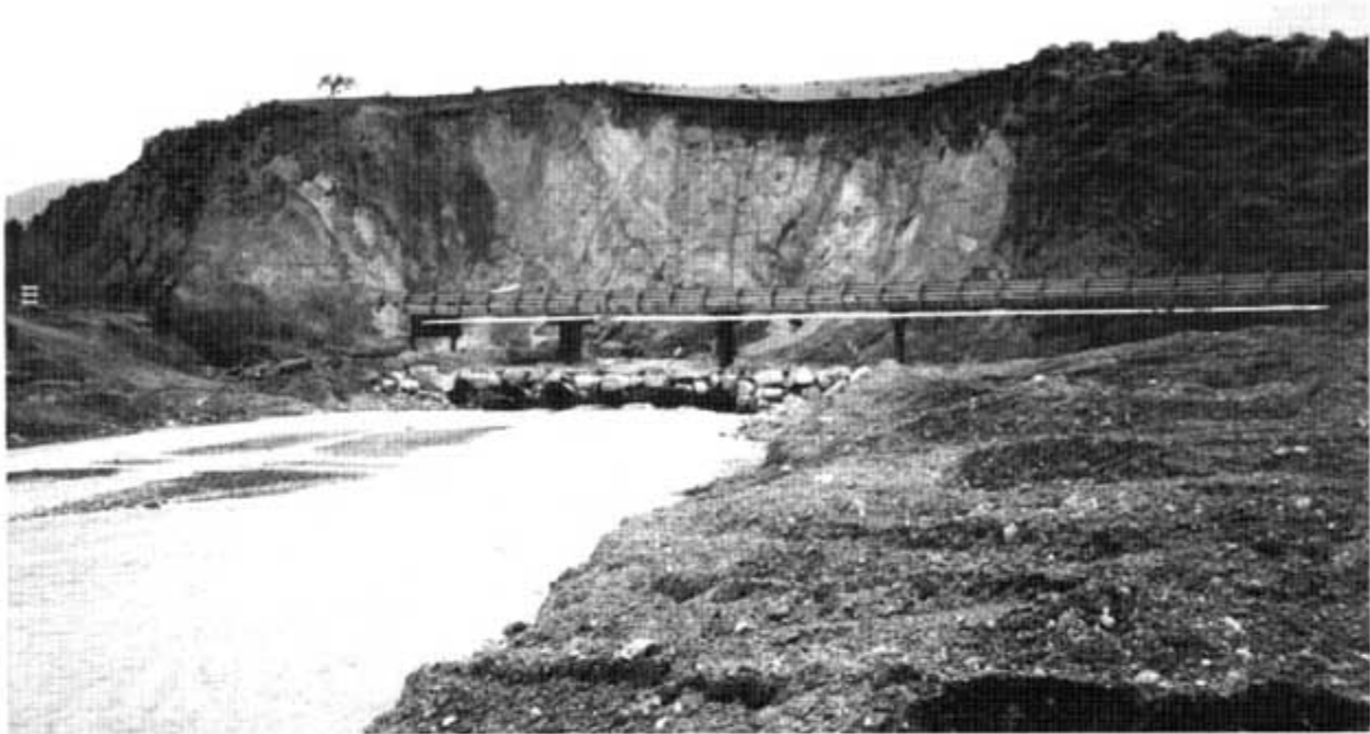
Figure 5. Graves Bridge after Jones Slide and flood of February 1998. The stream channel had been placed back under the bridge structure but the contractor had difficulty keeping the stream channel in this location. A substantial secondary landslide is visible behind the bridge.
