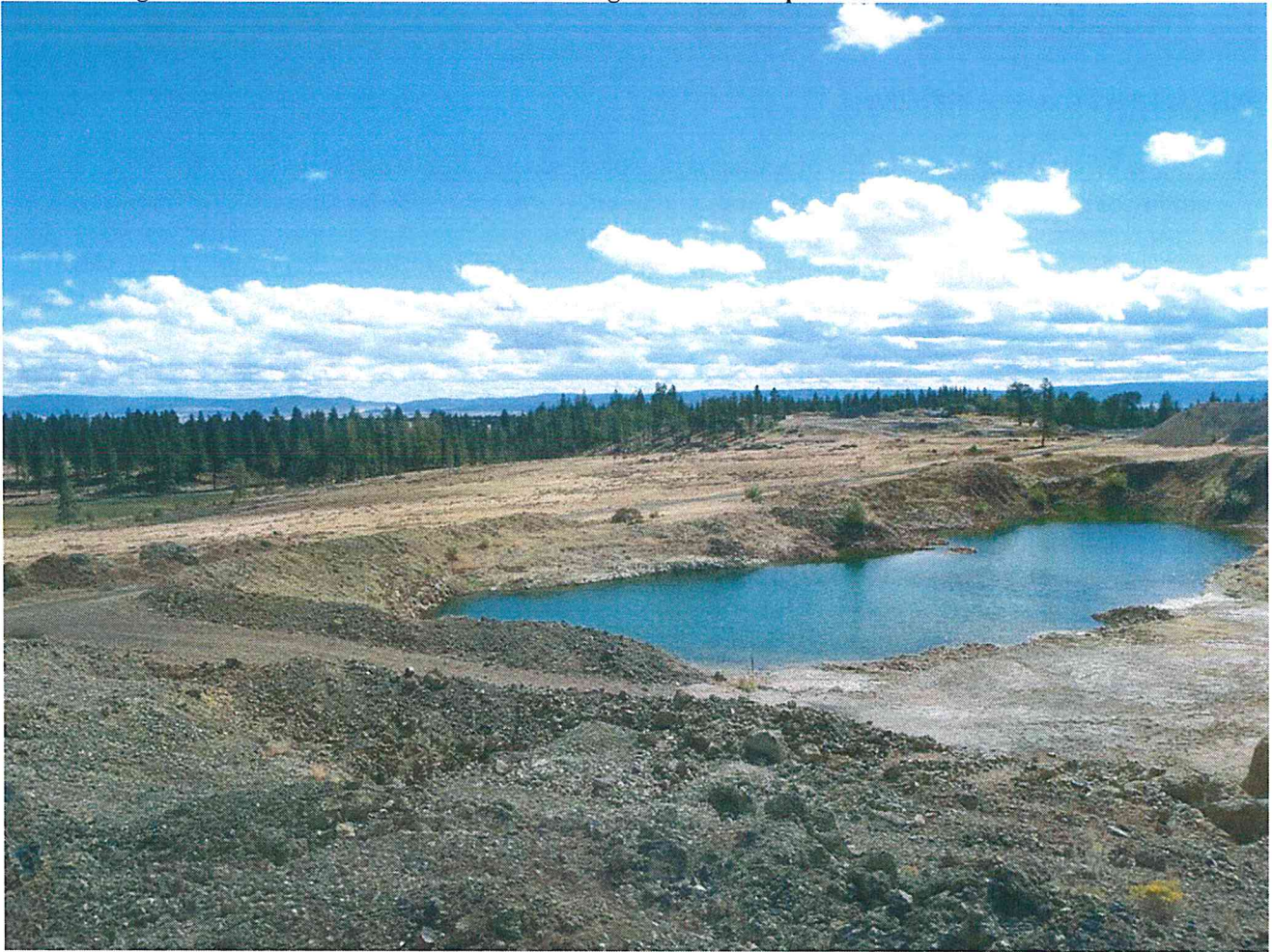
Photo 5: Large detention basins on the floor below the highwall shown in photo 4.
